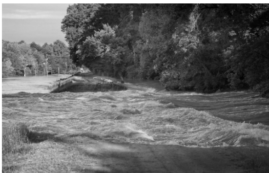
Figure 3. Levee breach (MTI)
