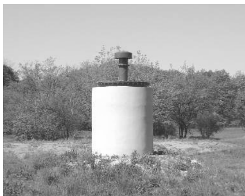
Figure 8. The aeration cylinder is raised above the flood level (Simon E.).
