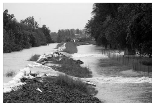
Figure 4. Overtopping the levee crest (MTI)
